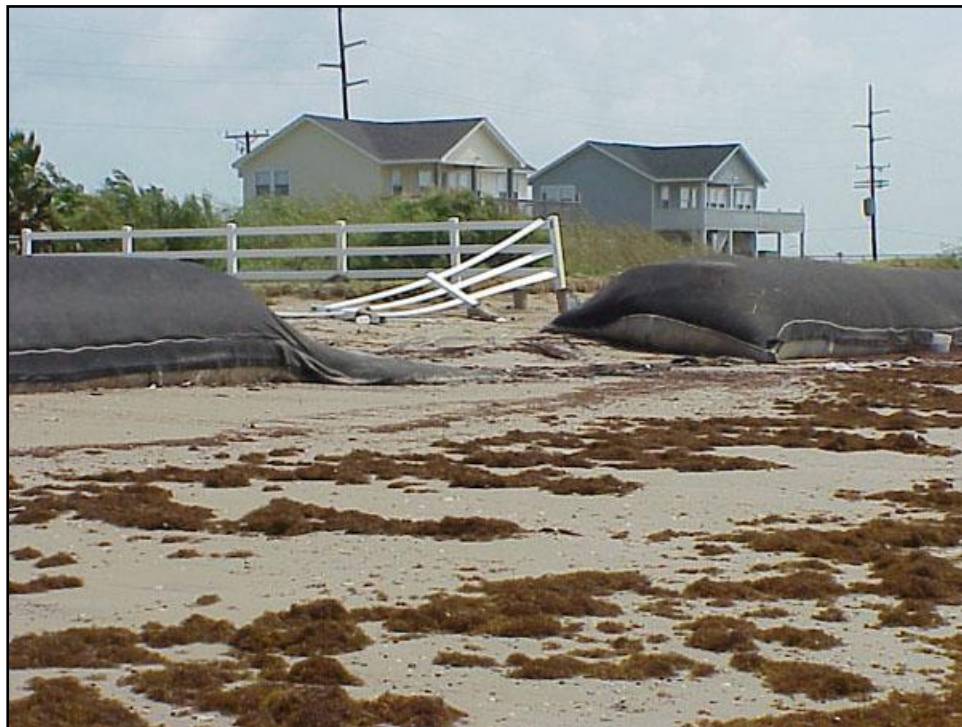
Figure 51. Hurricane Claudette induced localized geotextile tube damage on Bolivar Peninsula (2003). Photo courtesy of Shiner Moseley and Associates, Inc.
