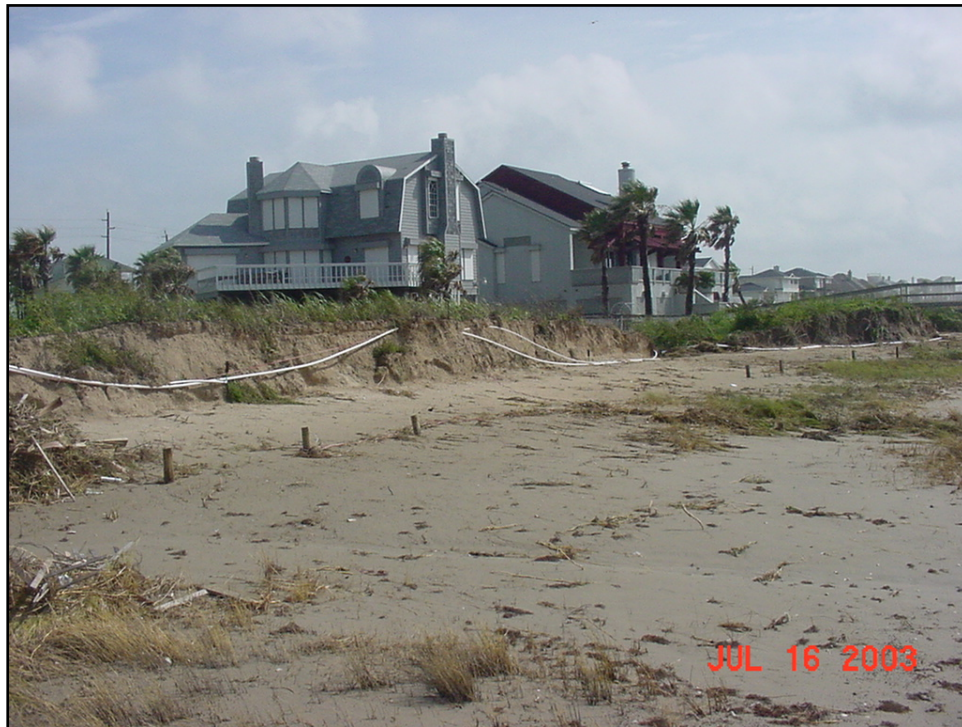
Figure 50. Berm and dune damage on Galveston Island due to Hurricane Claudette (2003). Photo courtesy of Galveston County.
