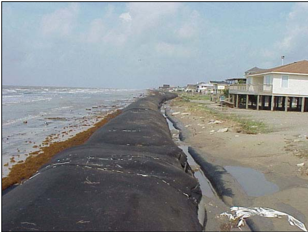
Figure 52. Bolivar Peninsula - Geotextile tube is fully exposed with minor erosion damage on landward side (2003). Photo courtesy of Shiner Moseley and Associates, Inc.
